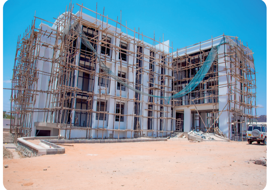
PPRA Headquarters building under construction, October, 2023
